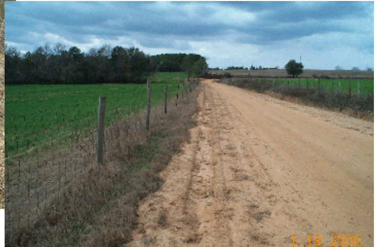
False ditch created by shoulder traffic and rutting
