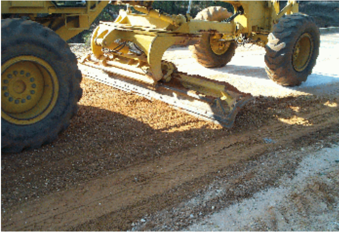
Proper moldboard forward tilt for blading.
