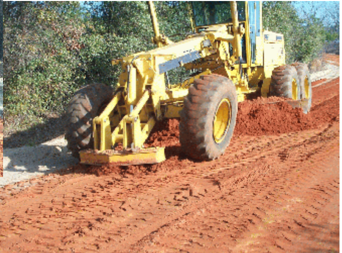
Clay blended into roadway surface with scarifier and blade
