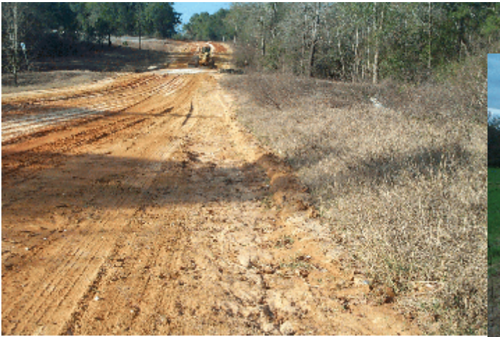
False ditch created by vegetal impediments
