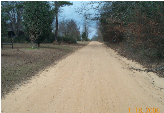
Exhibit 1.1b - Examples of 0" to 1/4" crown with no road ditches in place. Water infiltrates the soil of the sandy and flat road surface minimizing runoff from the roadway. The water that sheds from the roadway is readily removed from the road surface into the roadway edges allowing a passable lane in the center of the roadway.
