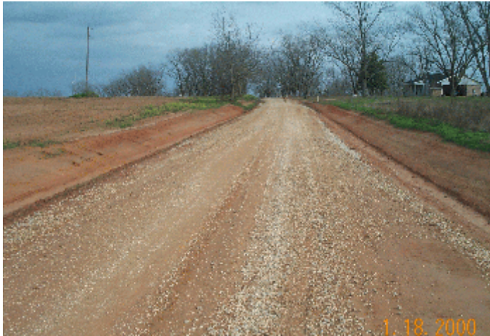
Exhibit 1.1a - Examples of 3/4" to 1' crown with road ditches in place. Water sheds readily off the crowned road surface and into the ditches. Proper drainage off the roadway surface helps to maintain a good "crust" which stabilizes the roadway and helps provide a good riding surface.
